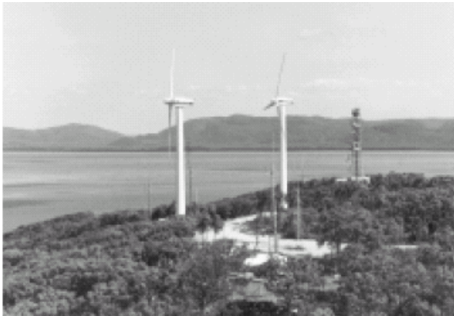
Thursday Island Wind Farm
