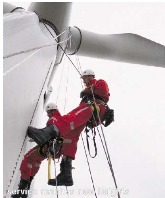
Routine Detailed Inspection of Blades
